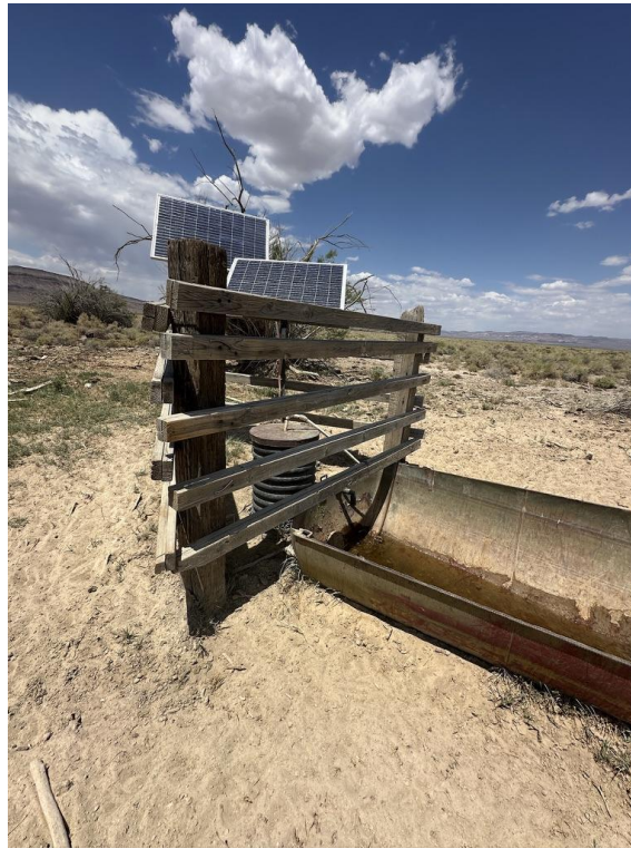
Fig. 35. A solar-powered well pump connected to a water trough, surrounded by signs of heavy grazing and trampling by cattle and feral equids.
