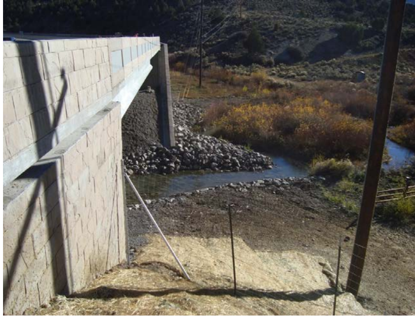
Figure 7. A second view of the Tucker wildlife bridge and culvert, completed early summer 2011 by Utah Department of Transportation. Photo courtesy of P. West, UDOT, used with permission.
