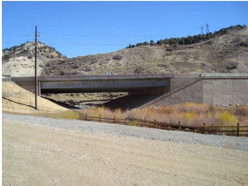
Figure 6. The newly constructed Tucker wildlife bridge and culvert. Photo courtesy of P. West, UDOT, used with permission.
