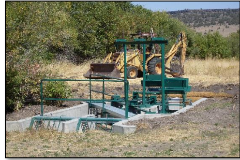
Figure 8-3. A roll drum fish screen located on the lower Taylor Diversion on Honey Creek.
