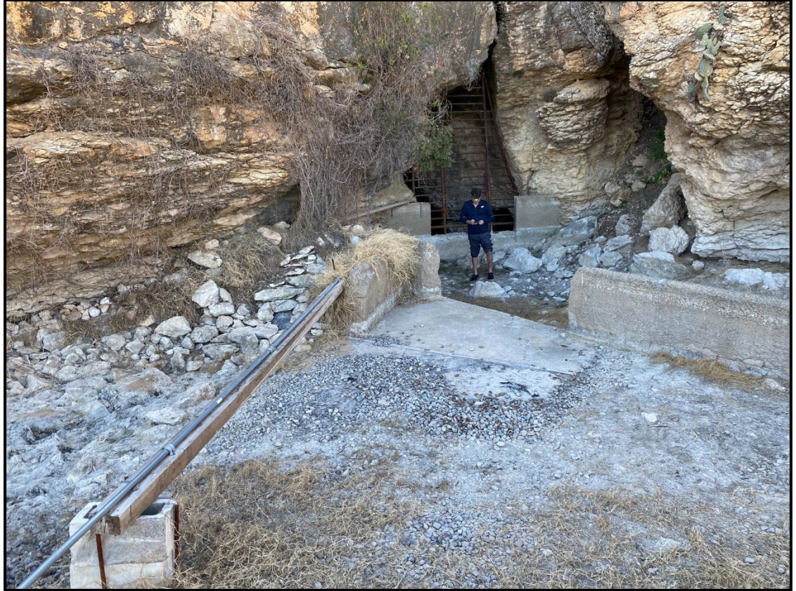
Figure 2. Dewatered Phantom Lake Spring ciénega (i.e., gray, barren area), February 2023. Individual in background stands in front of Phantom Spring Cave. Water no longer flows from the cave's entrance due to loss of pumped water. Image courtesy of Mike Montagne, Texas Fish and Wildlife Conservation Office.
